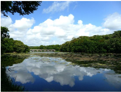
Eight Arch Bridge, Bosherton
